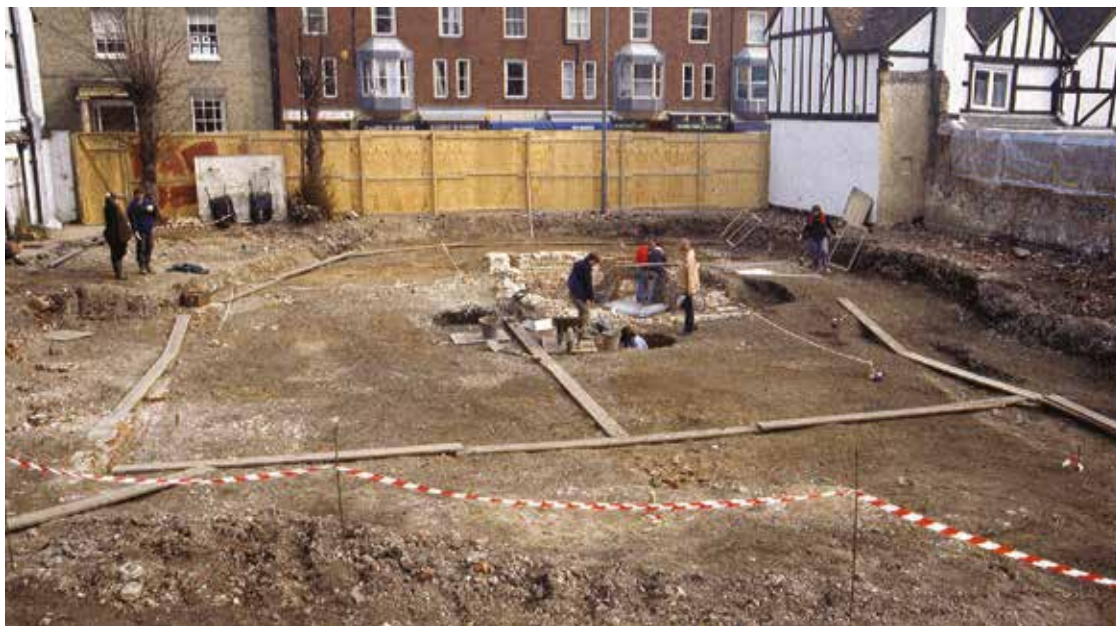
FIGURE 4 Overall view of site during the course of excavation, looking towards the High Street from the west
