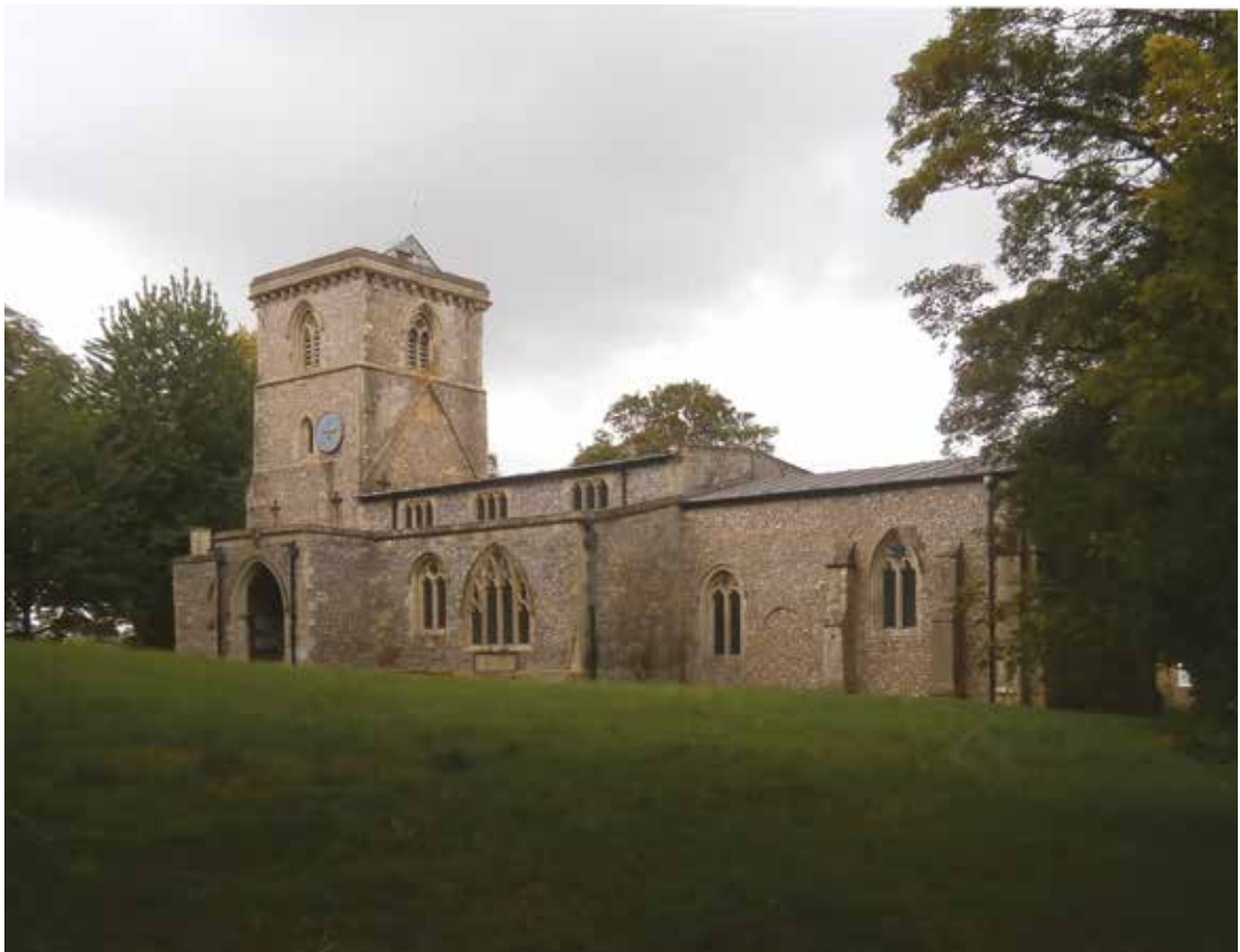
FIGURE 2 Bledlow, Holy Trinity Church, general view from south-east
