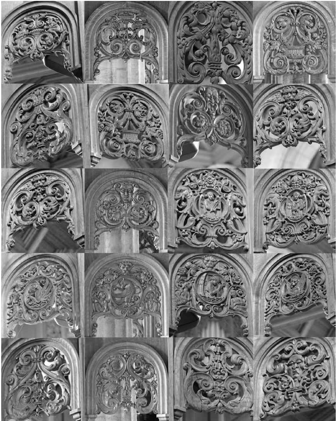
FIGURE 31 Openwork Infillings of the stall side arches
