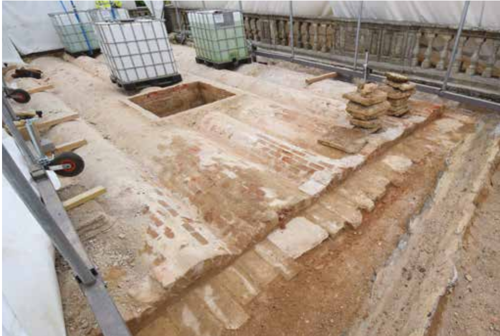
FIGURE 9 Brick vaulting and square base of former skylight exposed over eastern fernery
