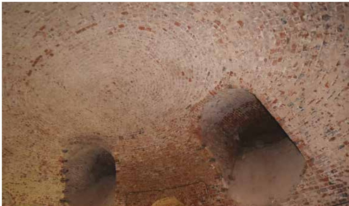
FIGURE 7 Light wells or funnels exposed within Sounding Chamber beneath mansion
