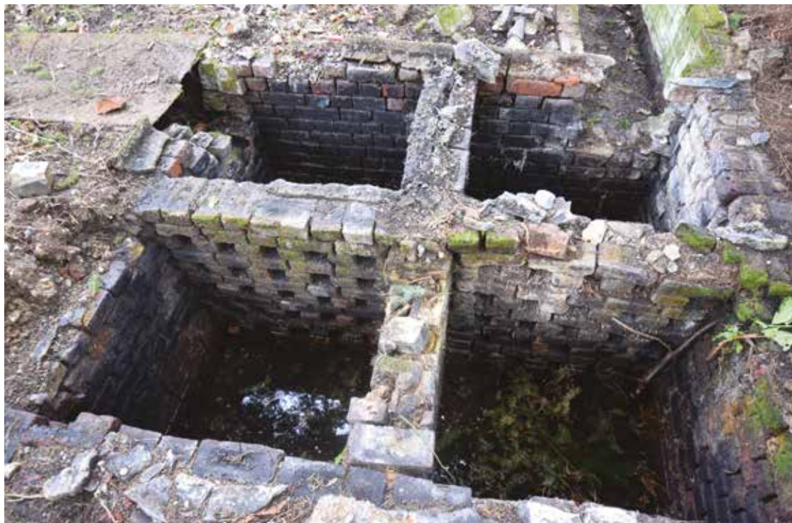
FIGURE 8 Brick-built silencing or condenser chambers outside the south-east corner of the generator house
