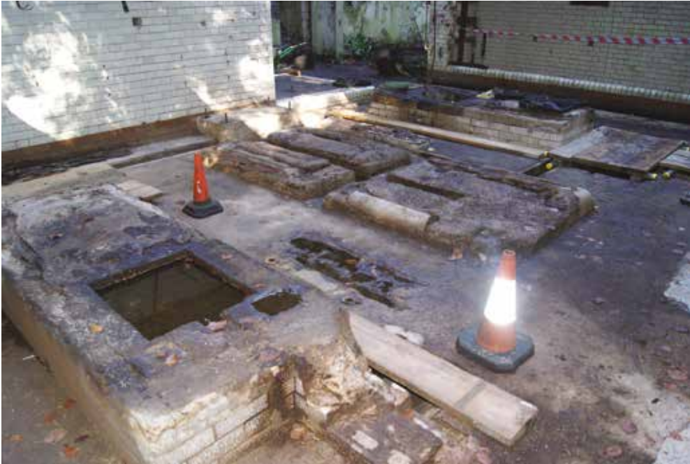
FIGURE 5 Engine bases looking north-west
