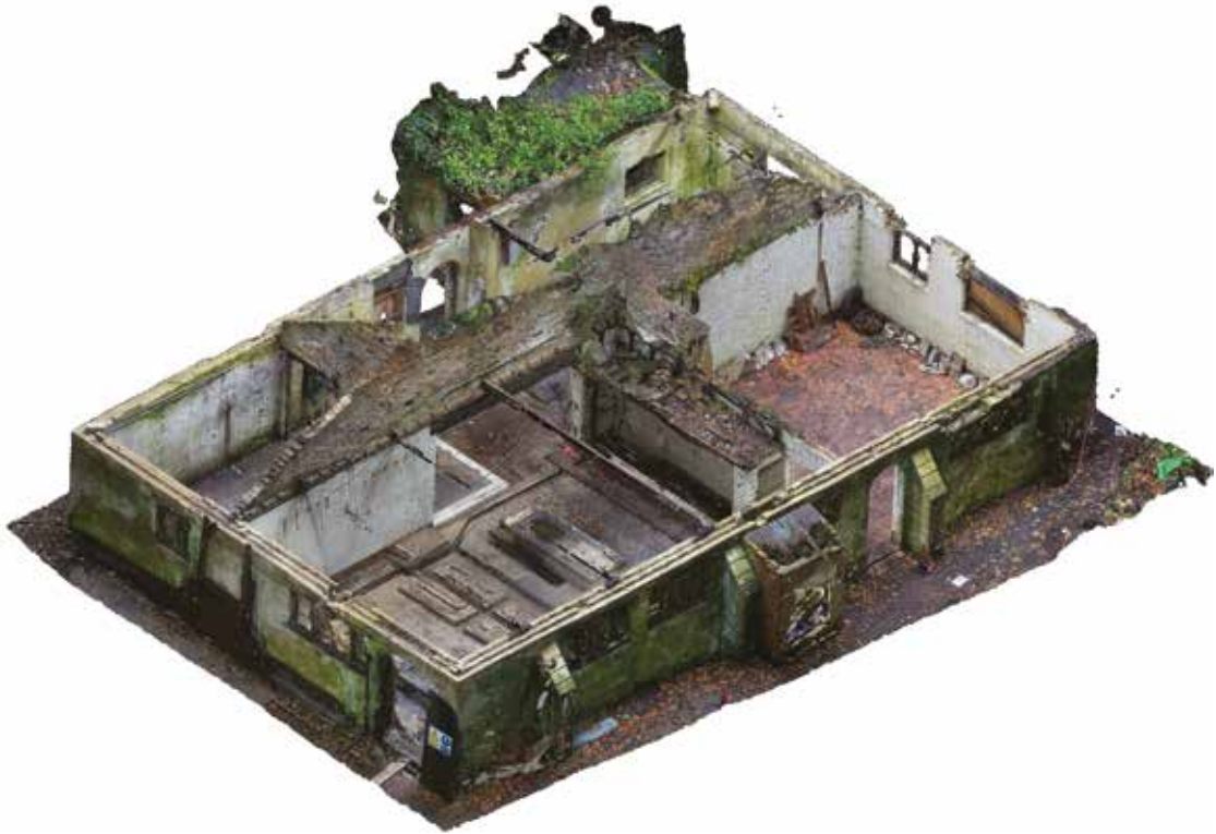
FIGURE 4 Bird's eye photogrammetric view of the generator house looking north
