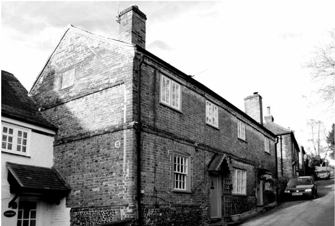
FIGURE 8 41 Church Lane, showing the front elevation added in the mid-18th century
