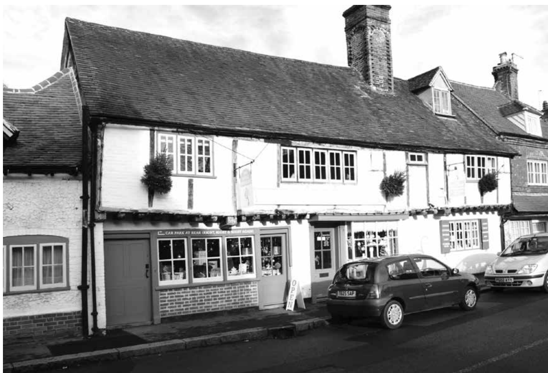
FIGURE 9 The Apple Orchard , illustrating the original jettied frontage dating from the first half of the 16th century
