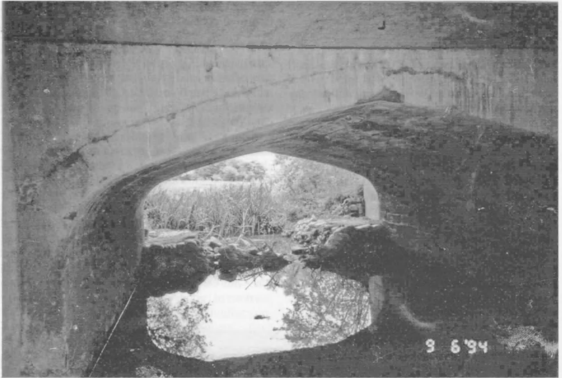
FIGURE 11 The arch of Hardwick bridge facing upstream. The lowest part of the reinforced platform lying on top of the bridge and also on side abutments are discernible. September 1994
