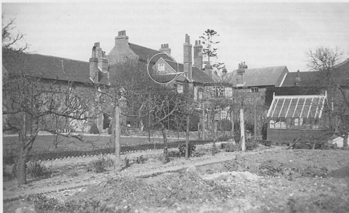
FIGURE 9 Latchmoor House (now Walpole House) with gable of the original house circled.
