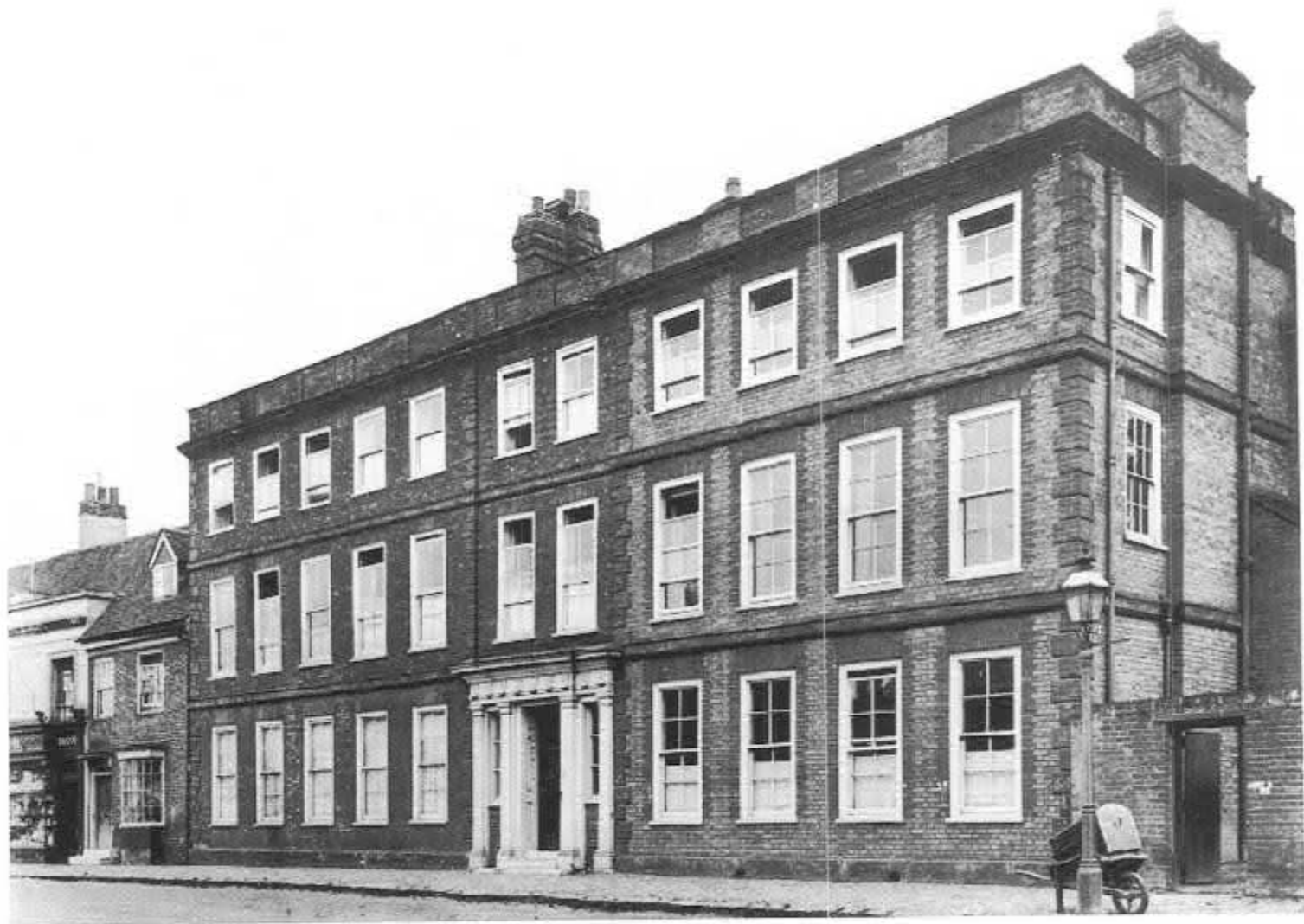
Fig. 10: Elmodesham House c. 1910, N elevation.
