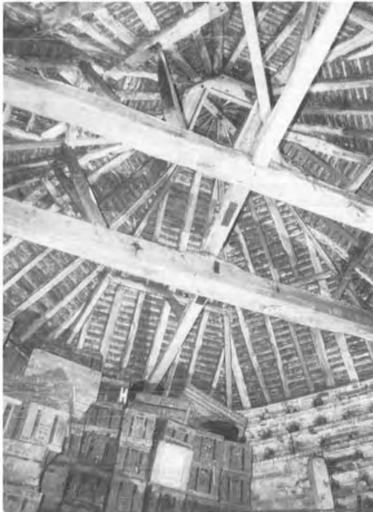
Figure 9. (below right) The roof structure and western walls above the inserted privy, showing the square aperture through which the pigeons entered. The axis of the former potence is at bottom right, and its upper bearing is at the Centre.
