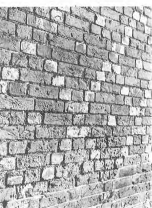
Figure 6. A section of the brickwork with the sun glinting on the vitrified blue bricks which form the diaper pattern. The nail-holes near the bottom indicate that fruit has been grown against the wall.
