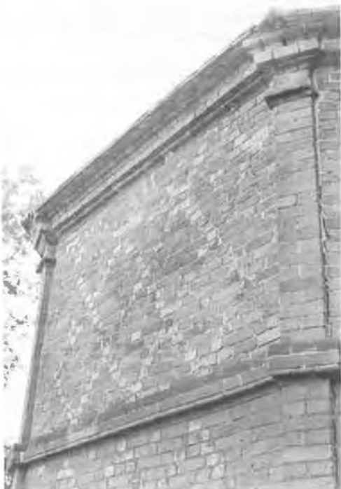
Figure 7. (below) The pilasters, capitals, eaves cornice, string course and diaper-patterned brickwork.
