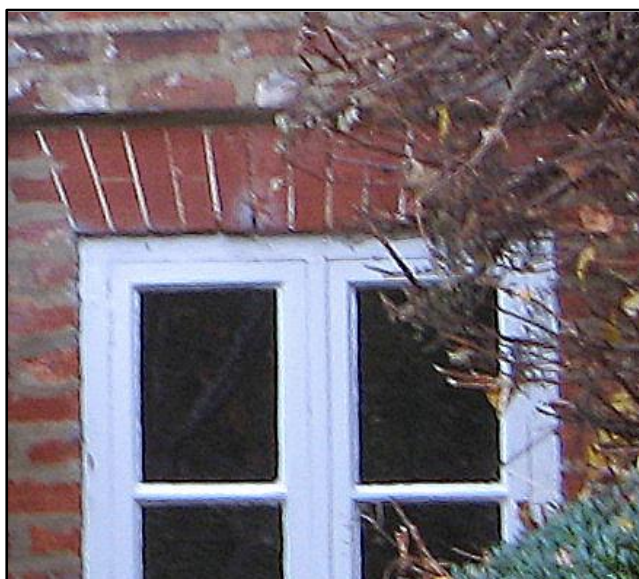
Figure 10: The finely-cut segmented brickwork over one of the windows.
