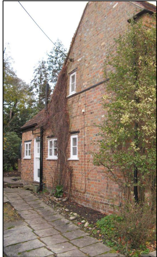
Figure 4: The north elevation. Note how the brickwork of the 1960s Kitchen extension on the left has been set to match the 1760s gable end.
