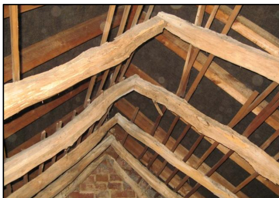
Figure 15: Old rafters left unused in the roof.
