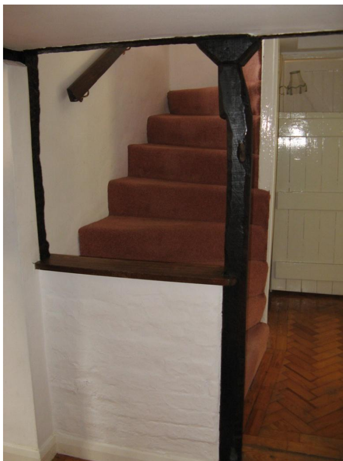
Figure 14: The 'winder' staircase, with recycled post.
