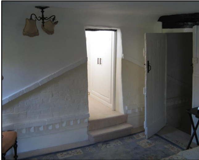
Figure 7: The 'internal pediment, cut by a later doorway.
